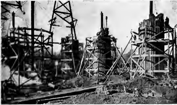
CYLINDERS ASSEMBLED FOR DRIVING
